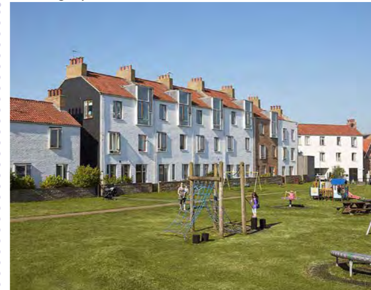
Example of landmark frontage to key open space, Southwold, by Ash Sakula Architects.
