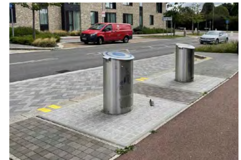
Underground refuse and recycling system, Eddington, Cambridge.
