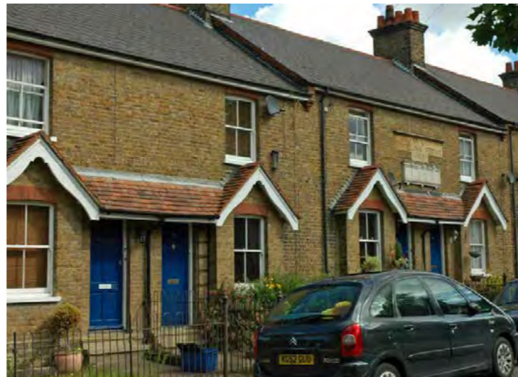
Articulated windows on Oddfellows Terrace, Old Harlow.
