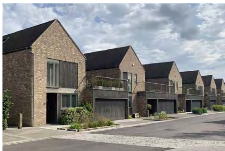
Well integrated enclosed car port with potential for future conversion to living space. Loveden Fields, Hampshire by John Pardey Associates.
