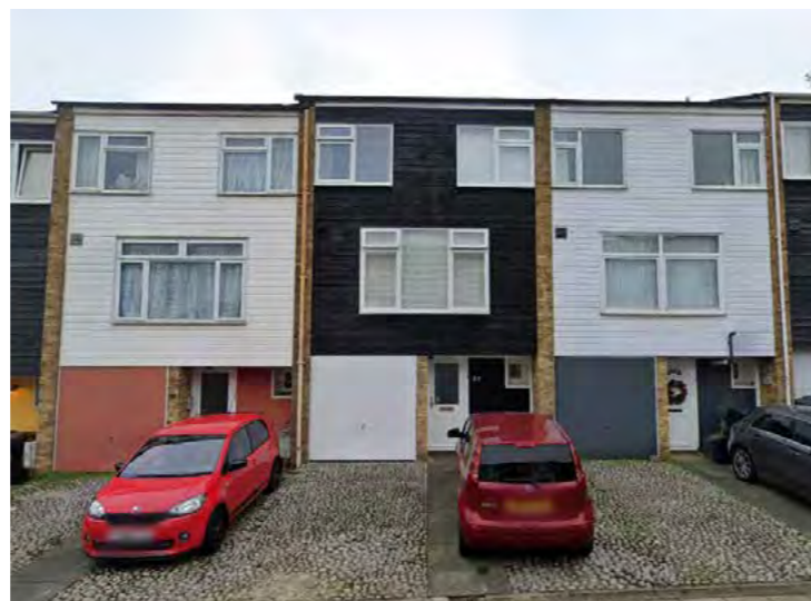
Strong composition and terraced rhythm at Morley Grove, Little Parndon, Harlow by Gibberd and partners.
