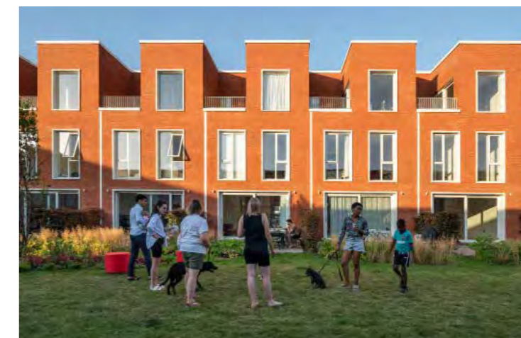
Broken terrace with terraces overlooking an open space. Brick House, Birmingham, by Glen Howells Architect
