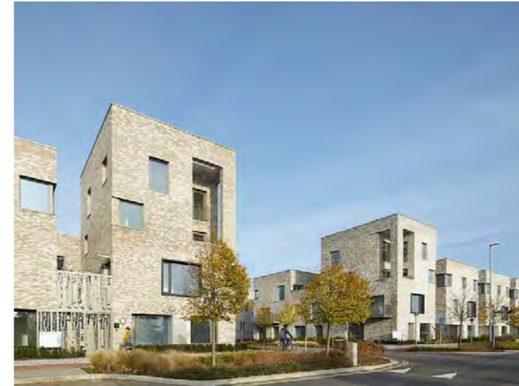
Grouping of buildings around a junction at Knights Park, Eddington, Cambridge by Pollard Thomas Edwards Architects.
