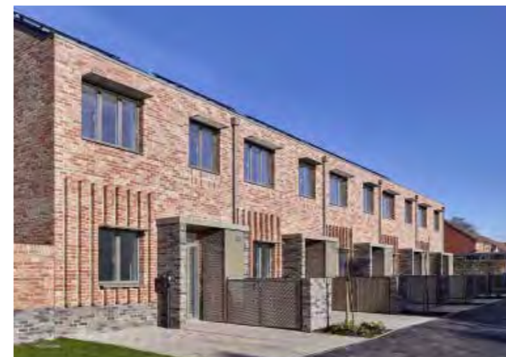
Considered bin enclosure design for terraced housing. Riverside Rd housing, Watford by Bell Phillips.
